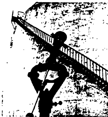
Spray nozzle for cooling outside of storage tank in case of fire.
