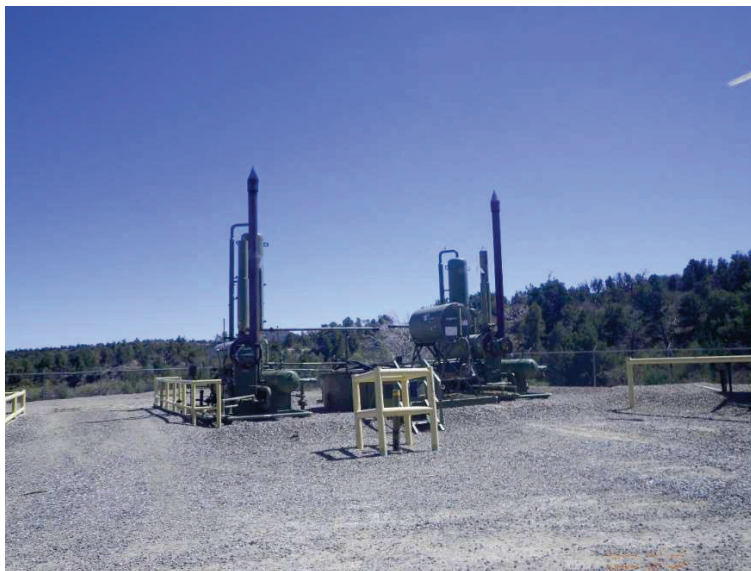
Image 6: Argenta Dehydrator #1 on right, Dehydrator #2 on left. RIMG0013.JPG
