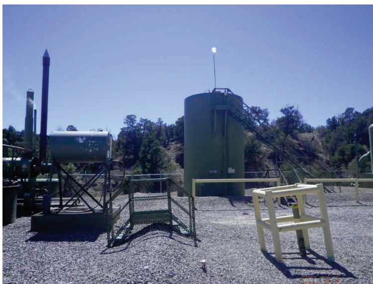
Image 5: Argenta produced water tank. RIMG0012.JPG
