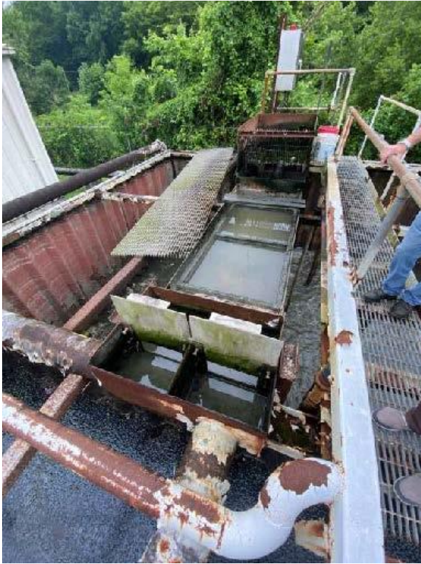
Figure 2: Photo of WWTP headworks
