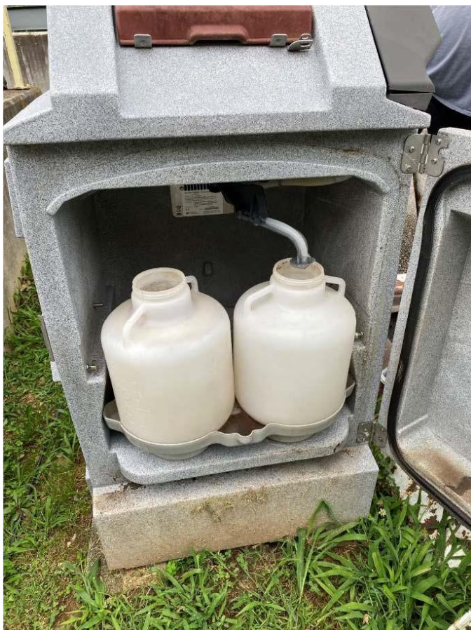
Figure 1: Photo of the effluent composite sampling unit that appeared to have not been used recently.
