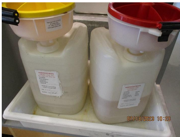
Photo 8: Chemistry Laboratory: Each bay contains a 5-gallon SAA for non-halogenated solvent waste (containers with red colored lids) and halogenated solvent waste (containers with yellow-colored lids). Each bay also has a 20-gallon red container for flammable, toxic solids.
