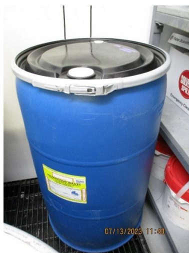
Photo 19: 55-gallon hazardous waste containers in the CAA. Containers are labeled, dated, closed, and marked with the indication of the hazard of the contents.
