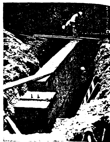
This pier carries the balances and is separate from the building structure.
