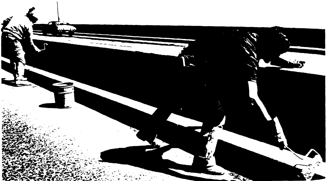
TBTA maintenance crew applies coating of lead-based paint to roadway center divider of Throggs Neck Bridge.
