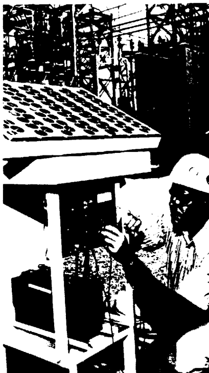
Solar-powered rectifier feeds 30 watts at 6 volts d-c to 15kv underground cable to minimize galvanic corrosion.
