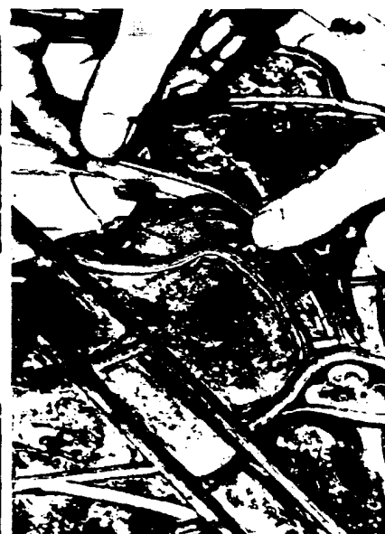
Restored Canterbury stained glass is reassembled and joined with ancient recycled lead.
