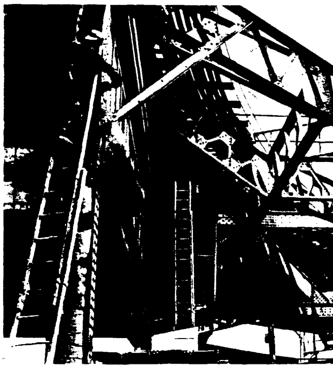
Lead-based paint is applied to part of structural steel that supports subway's elevated system.
