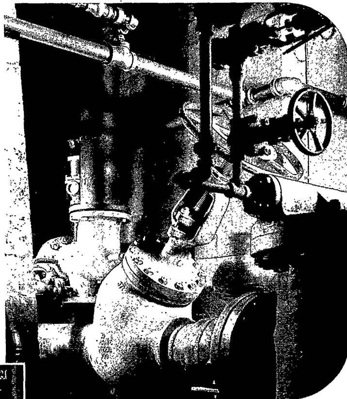
A Crane cast steel stop-check valve with butt-welding ends, and Crane forged steel valves, fittings, and unions in the power plant of a city railway.
