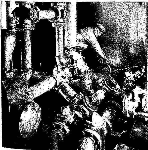
Crane Cocks in an intricate pumping system.
