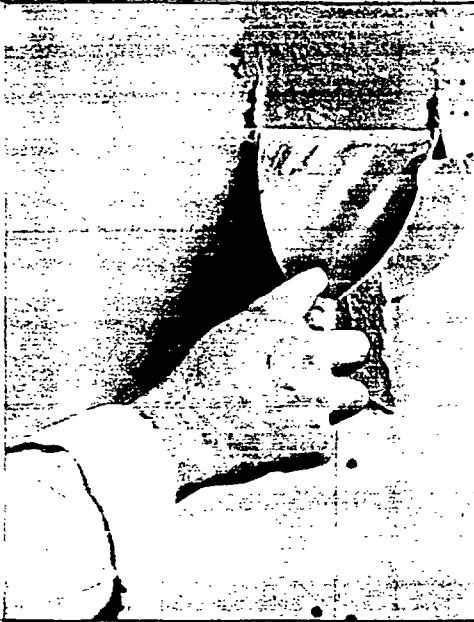
First step in Perf-A-Tape joint treatment: "Buttering" the Sheetrock joint with Perf-A-Tape Cement.
