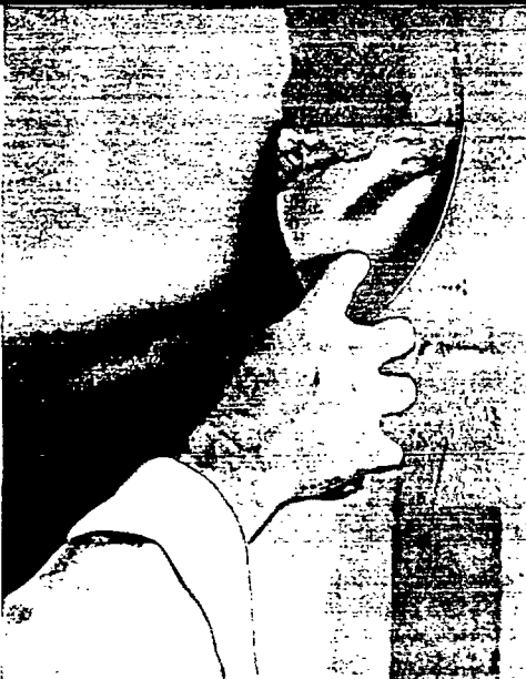
Applying cement over Perf-A-Tape, leveling surface and feathering edges to produce smooth, level joint.
