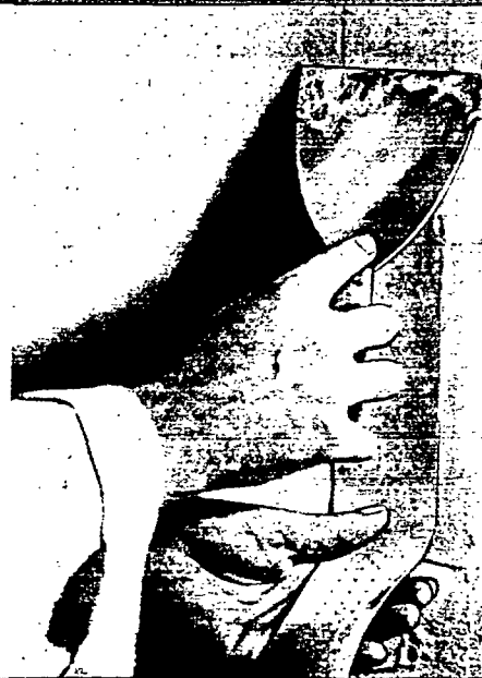
Forcing cement through perforations and leveling the face of Perf-A-Tape strip centered over joint.
