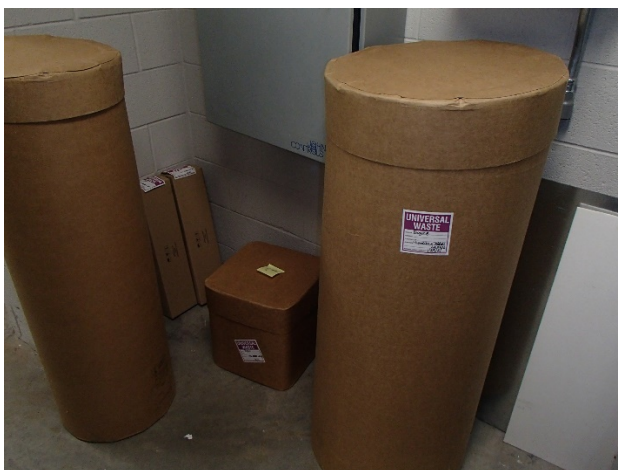
Photo 3: Room 24104 - Electrical – Universal Waste storage.
