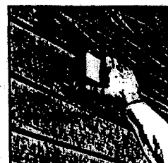
Before repainting a home the wood siding should be carefully prepared. Where the paint has scaled, a wire brush should be used to clean up the surface.
