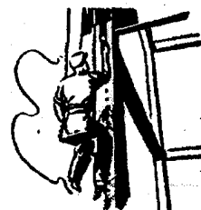
To guard against rust and corrosion, all exposed metal surfaces should be given a protective coating that weathers well.
