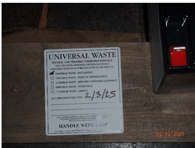
Picture 30 – Service Management UW Batteries label
