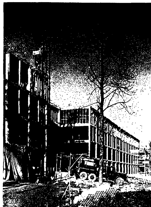
Buck Hoistowers in pits speed construction of the operations office building for the Government Employee Insurance Company of Bethesda, Maryland.
