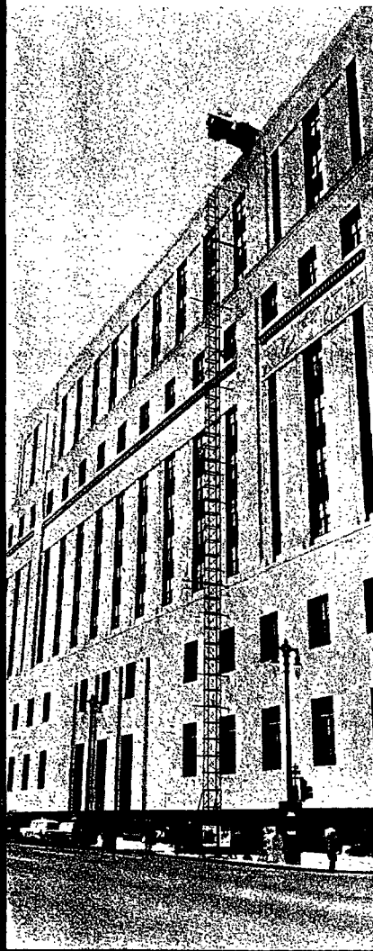
Roofing materials are hoisted to a 174 foot high take off point.
