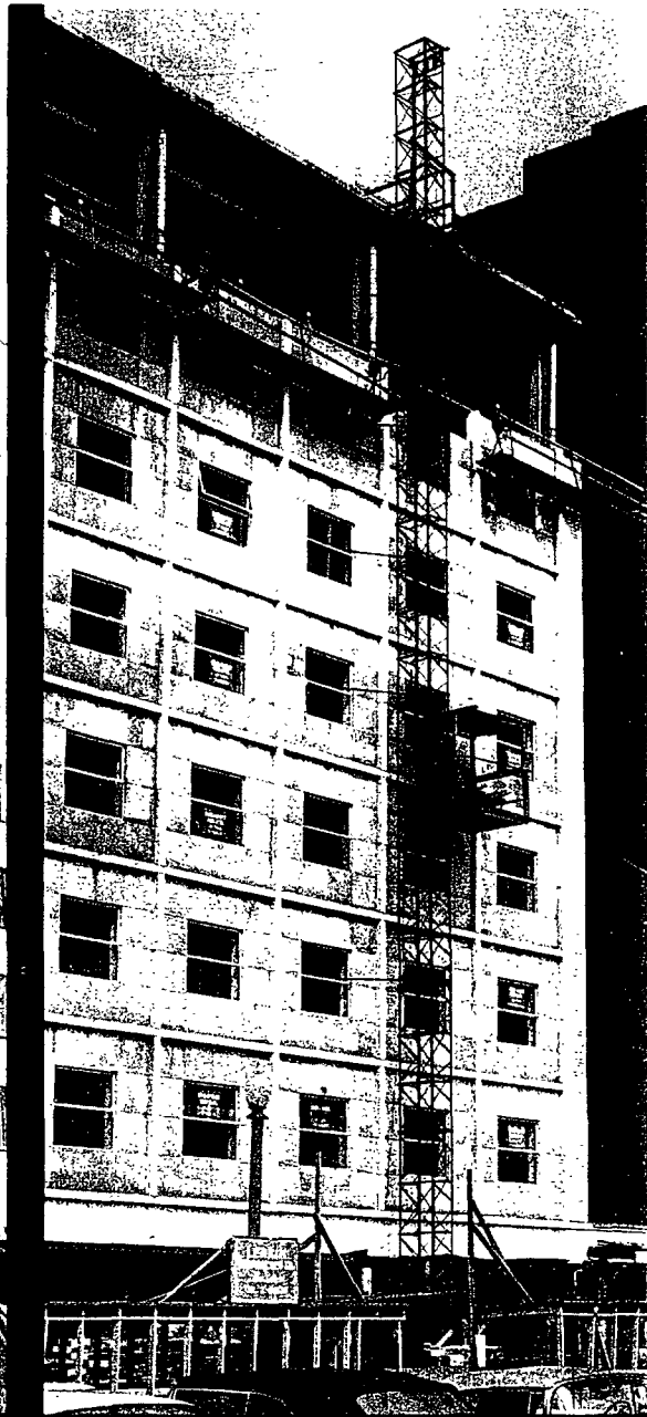
This 90 ft. high installation was put up by two men in one day.
