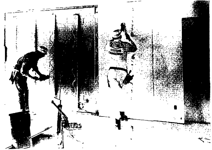
Completion of partition
