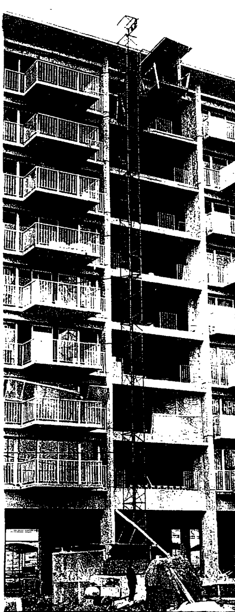
Dry wall goes up 6 stories on a special raised extended platform.
