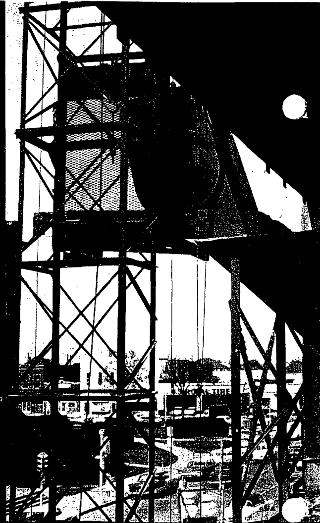
Concrete is dumped smoothly, automatically, on the second floor.
