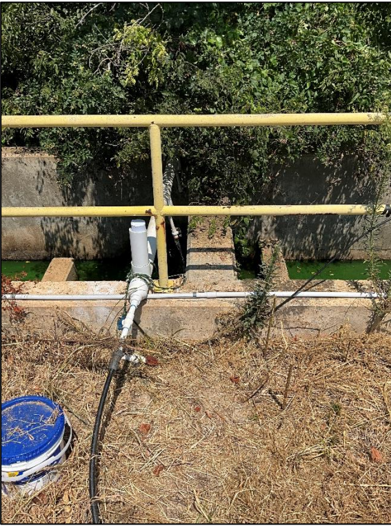
Photo 1: Chlorine tablet injection point.
