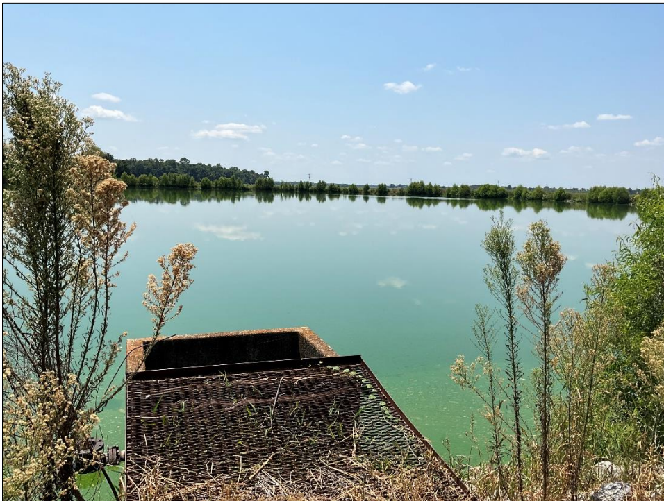
Photo 3: Crenshaw lagoon and berm.
