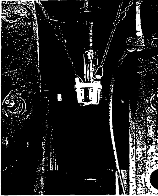
FIG 33-15 — Safety basket, made of 2 by \frac{1}{4} in welded steel, holds the piston rod of a forging hammer when the steam is shut off for cleaning ram bore. The ends of the bars are bent around the chain eyes
