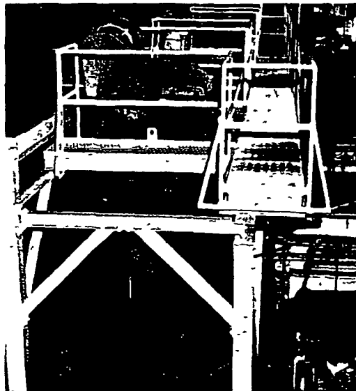
FIG 33-16 — Permanent catwalk installed along row of board drop hammers makes repair and servicing of hammers easy and safe
