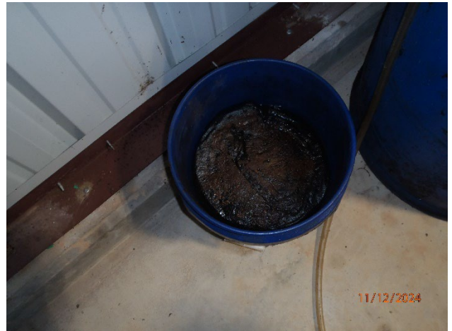
Picture 35 – E15 Building Used Oil and debris in container
