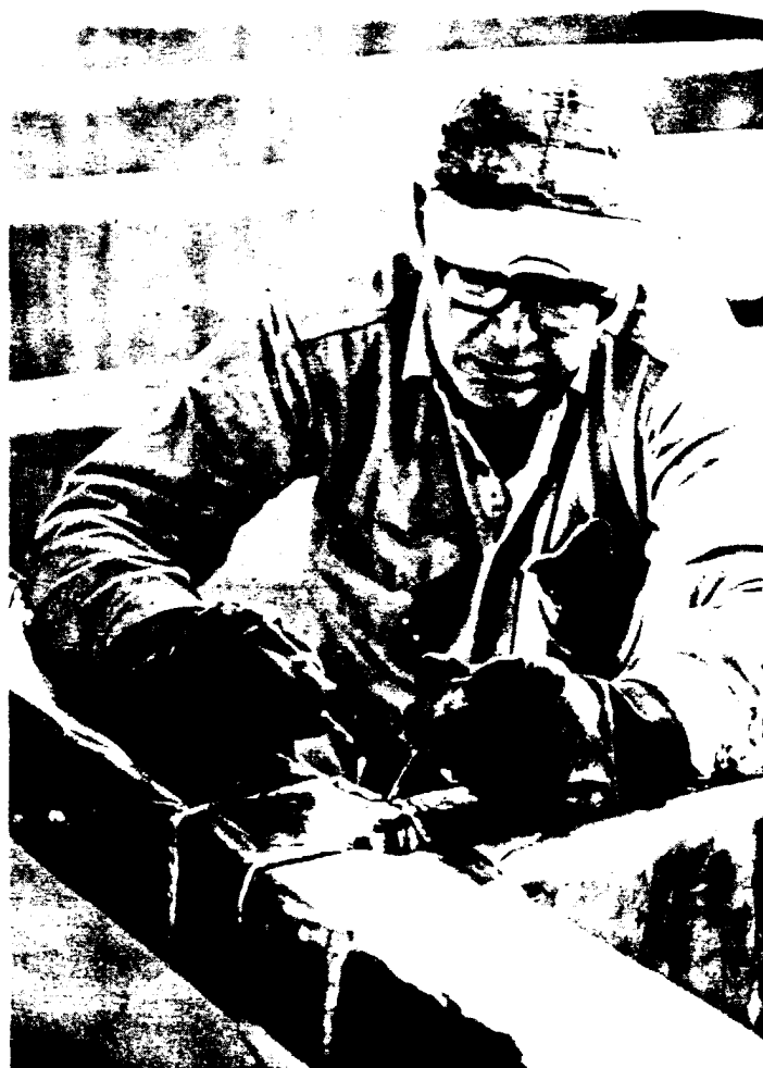
A fine-tipped torch is used to burn the corner seam of one of the refining tanks.
