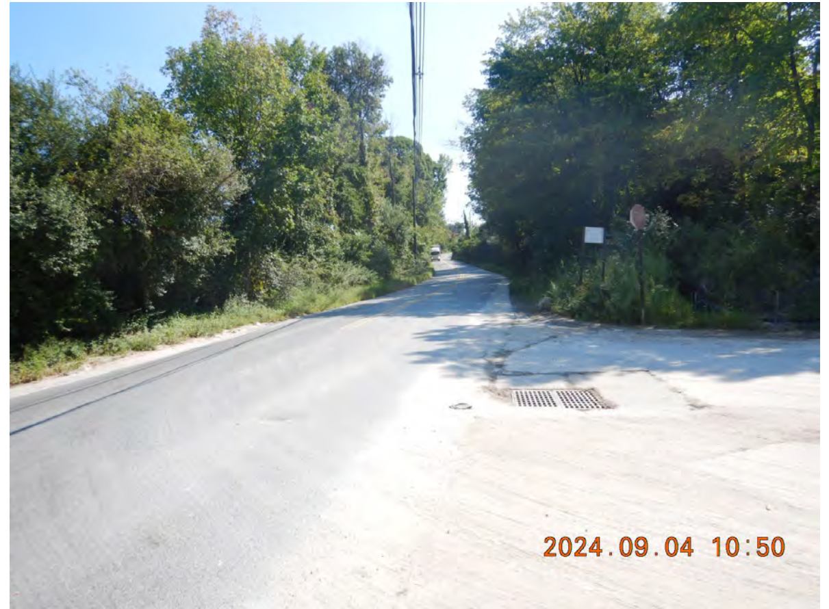
DSCN3767 – Catch basin near entrance; source material along road and driveway
