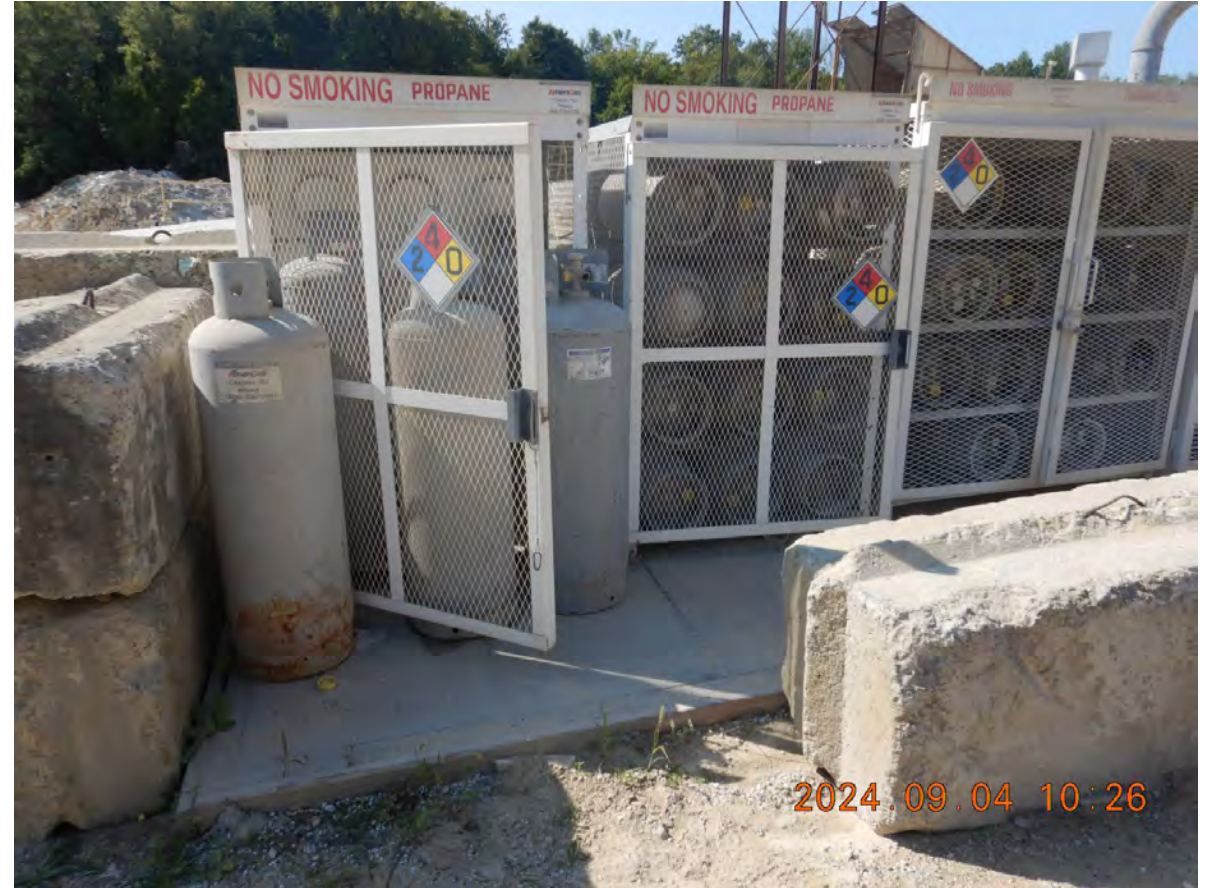
DSCN3749 – Propane canister storage; central area of Site
