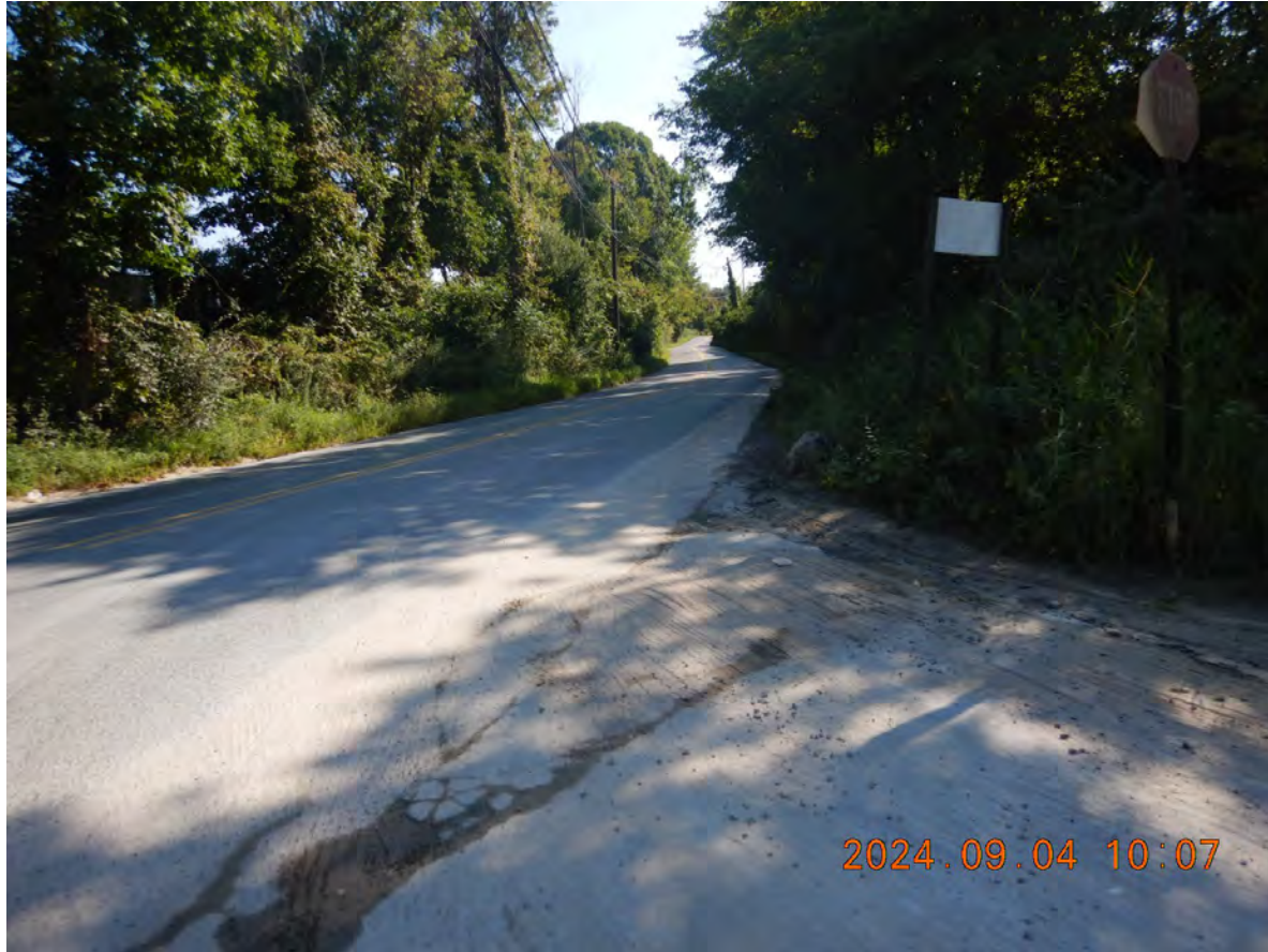
DSCN3691 – Source material tracked out onto Gold Mine Rd looking east
