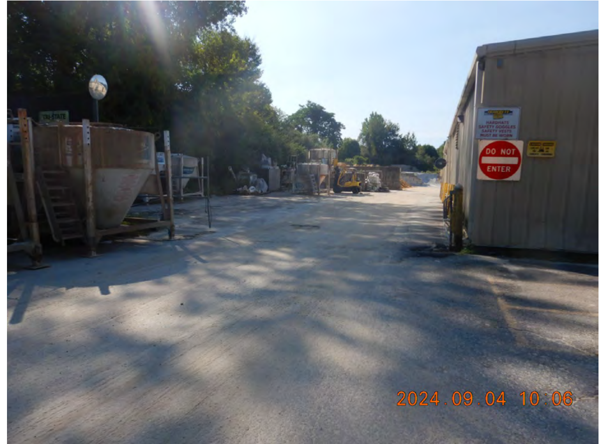
DSCN3683 – East driveway looking south toward aggregate bunks
