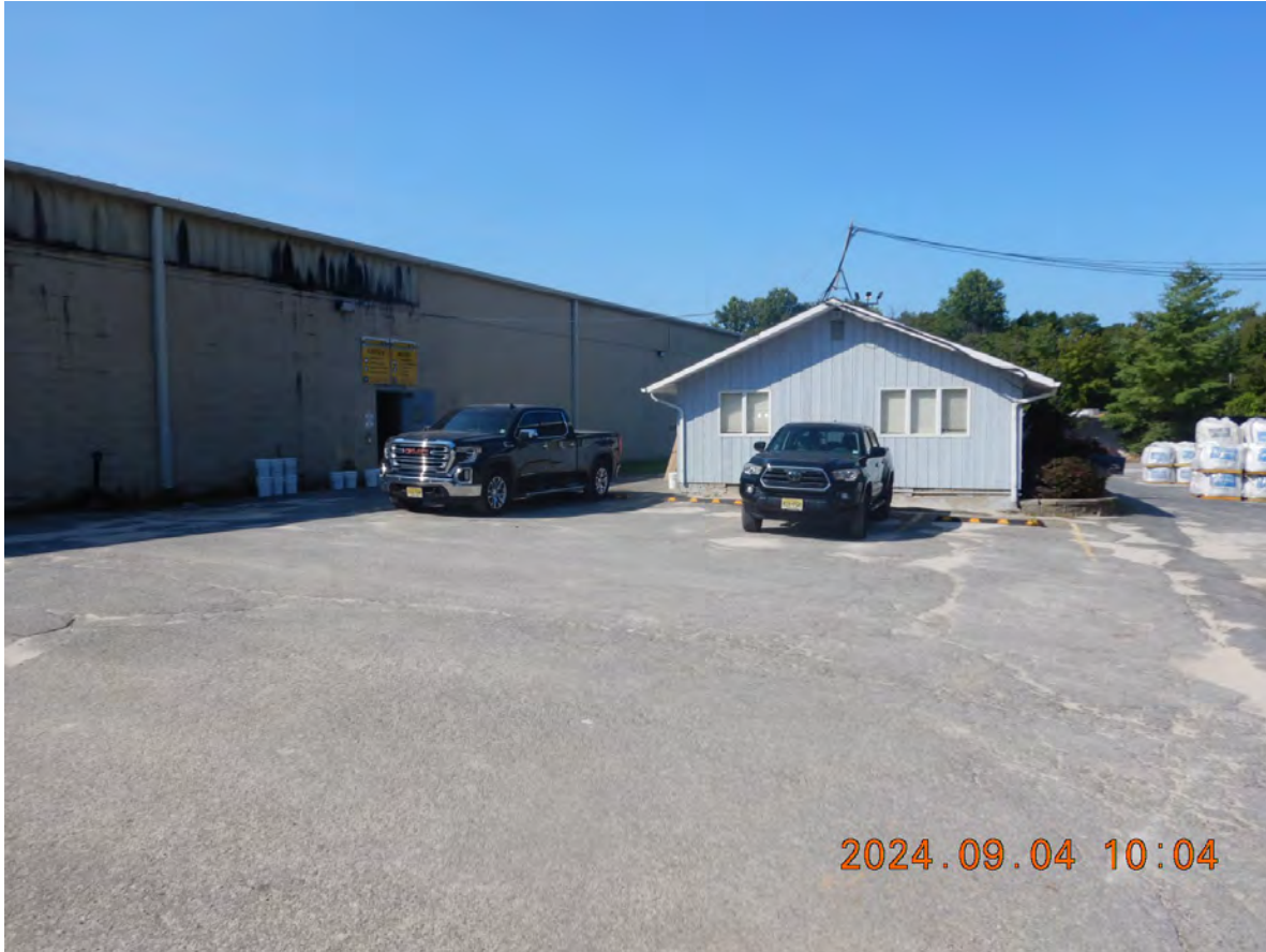
DSCN3680 – Office building on the northwest side of the Site
