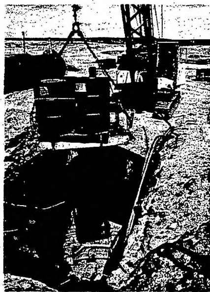
Storing chemicals in Idaho missile silo
