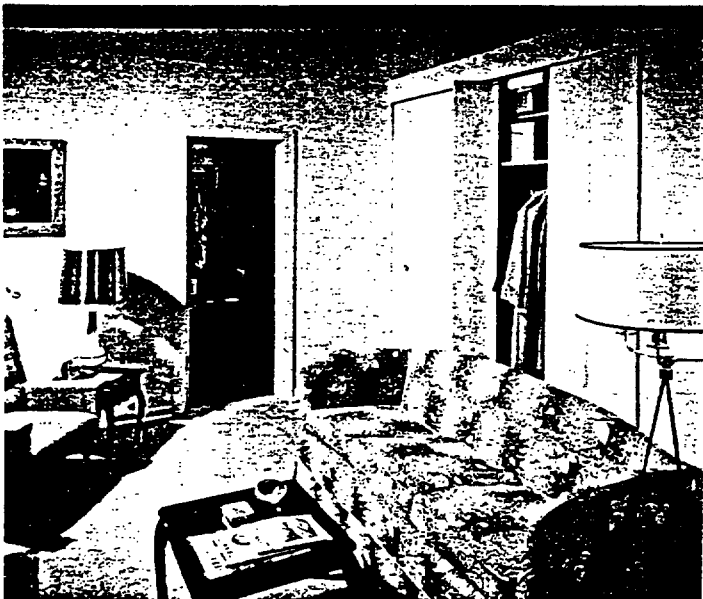
A PIPE CHANNEL to the second floor gave depth to this new partition which creates a closet when closed with doors.
