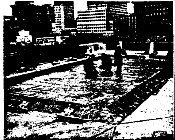
The rooftop pool, showing the 8-lb. lead lining and the lead apron extending around it.
