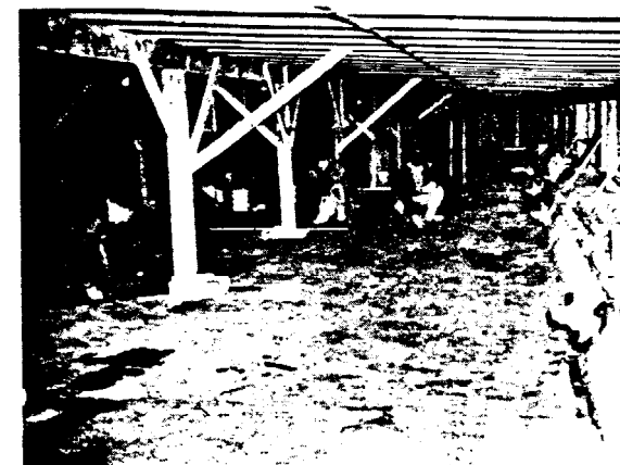
Lead burner forming a corner seam near a drain in the Plaza pool, the largest of its kind in New York. The area is covered by a temporary roof.
