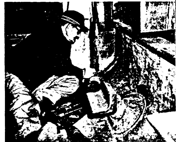
Lead burner forming a corner seam near a drain in the Plaza pool, the largest of its kind in New York. The area is covered by a temporary roof.
