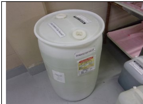
Figure 3: 10:22 AM Acid Storage (Photo 2 of 2) One of two 35-gallon containers observed with hazardous waste label, accumulation start date, and indication of the hazards of the contents.
