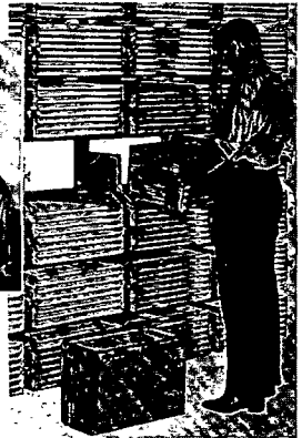
KOMPAK Servicing operation consumes at the most 3 min. per unit—unloading, refilling and replacing. Life of filter medium varies from 3 to 6 months depending on dust content of the air.
