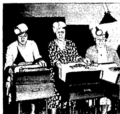
Courtesy Mine Safety Appliances Co. The electric lights were dead but this bank continued to serve its patrons with the aid of miners' cap lamps.
