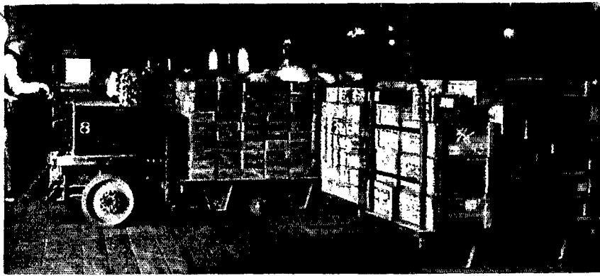
Method of stowing freight on skids in pier warehouse.
