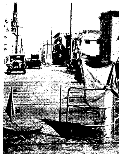
Wind sails for use in street manhole ventilation.
