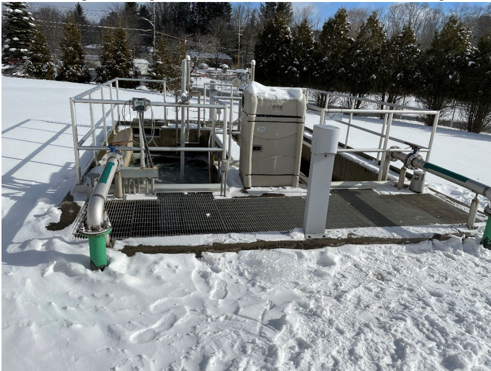
Photo #2. 6-Hour composite sample was collected from the effluent monitoring location.
