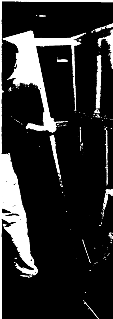
Lead acoustic panels can be readily installed by one man without mechanical help.
