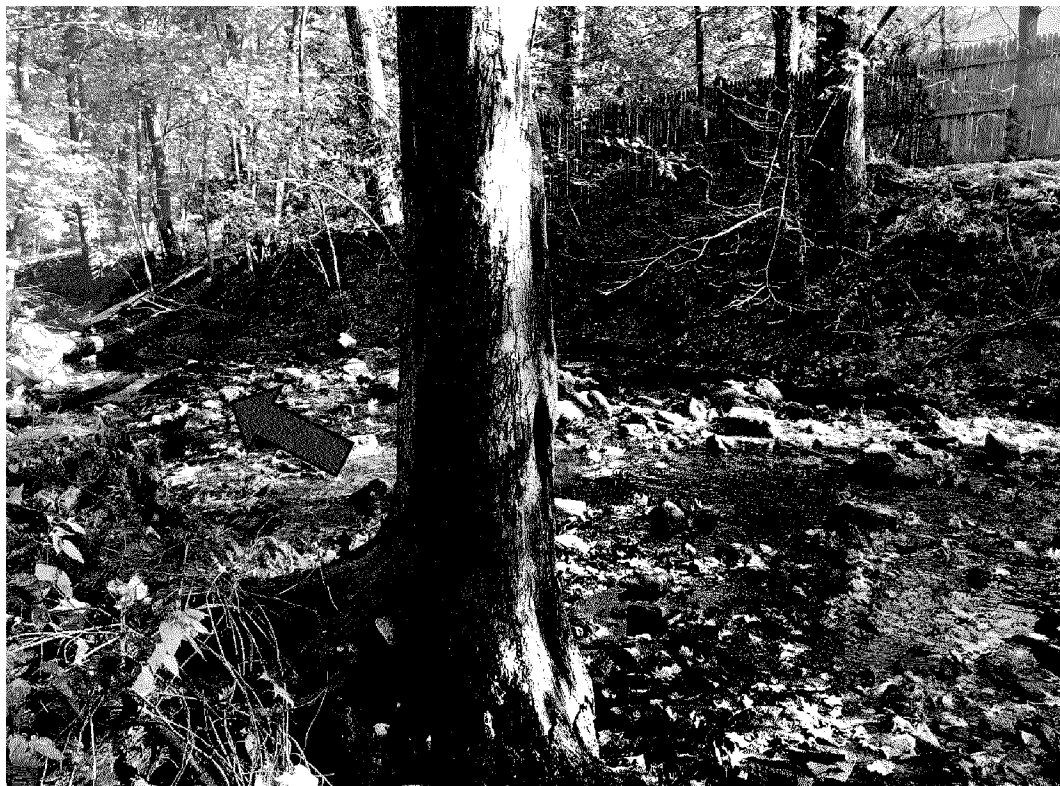
FitzCoburn2: Fitzgerald Brook downstream of street culvert. Flow direction indicated by a blue arrow.
