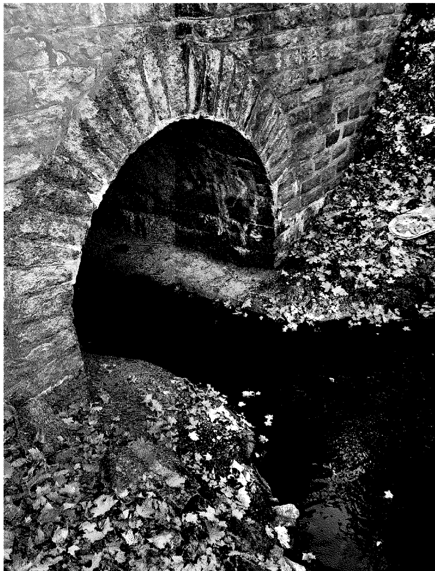
FitzLakeAve1: Fitzgerald Brook street culvert located on Lake Avenue near the intersection with Anna St. Sample location indicated by a red X. Flow direction indicated by a blue arrow.
