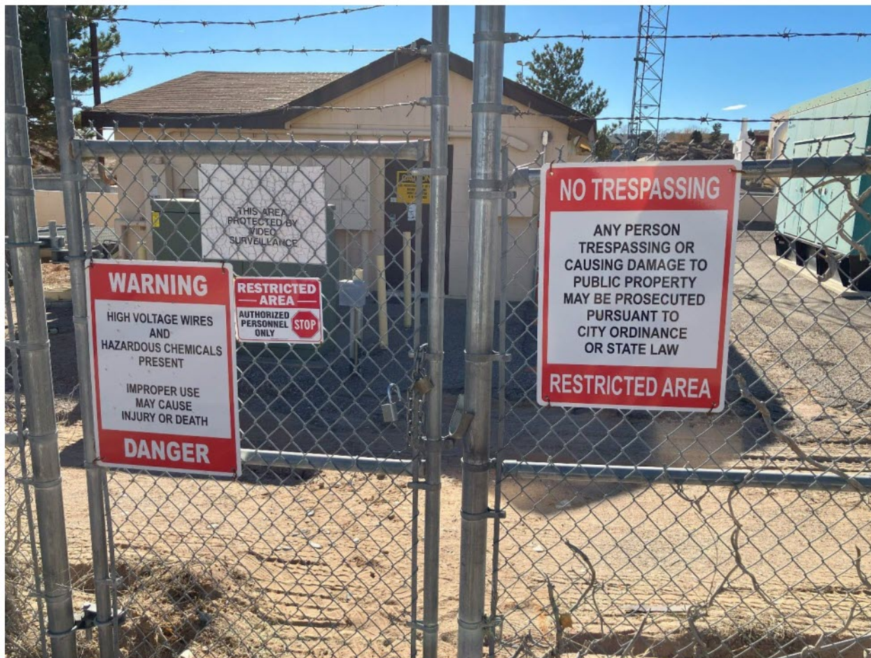
View of warning signage on outside of WWTP #3 and LS-#21 wire fabric perimeter fencing. (IMG_0456) Photographed by N. Fuad
