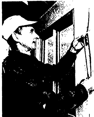
Cut-off strips are removed. The overlapped right hand flap that was cut is pulled out from under the left flap.
