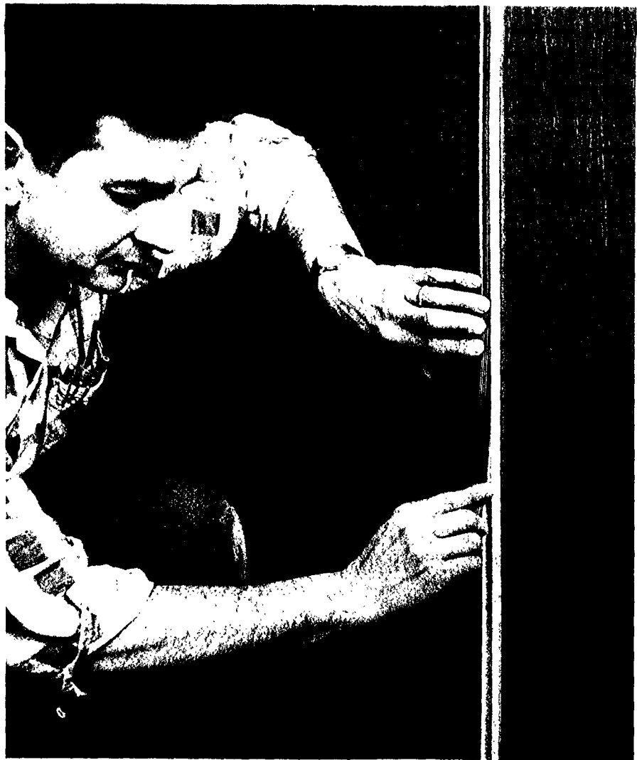
Fig. 64 Screws holding predecorated wallboard are concealed with vinyl strips in battens which cover joints.
