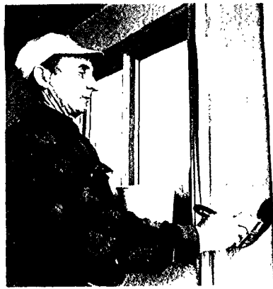
When the joint compound sets, the area is coated with wheat paste.
