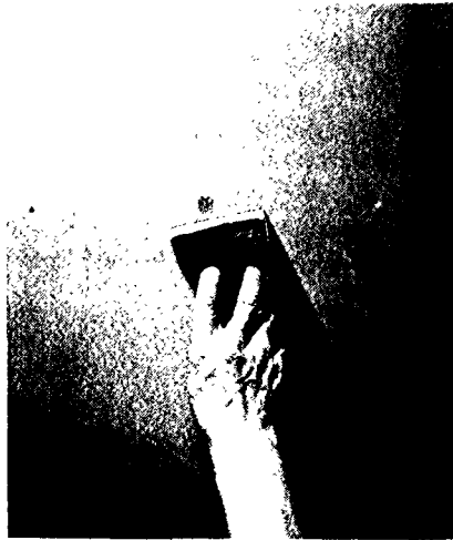
Fig 62 The dimpled depressions from fasteners must be treated with compound before gypsumboard is decorated. More than one coat is often necessary.
