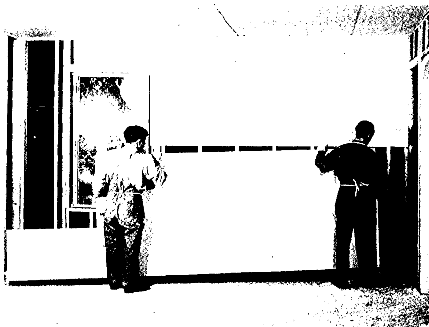
Fig. 15 Gypsumboard applied horizontally provides a stiffer surface finish. Measurements at each corner of framing and gypsumboard must be made carefully to assure close fit around openings.
