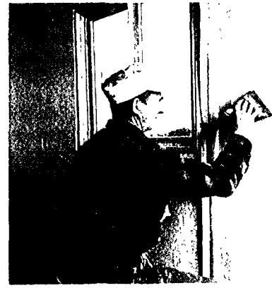
The right hand flap is pasted down and smoothed; then the left flap is pasted over the right hand flap.
