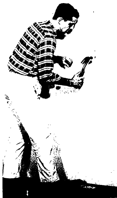
Fig. 33 Gypsumboard applicator lifts board into place with a foot lever and leans against board with his forearm to hold it firmly while nailing.
