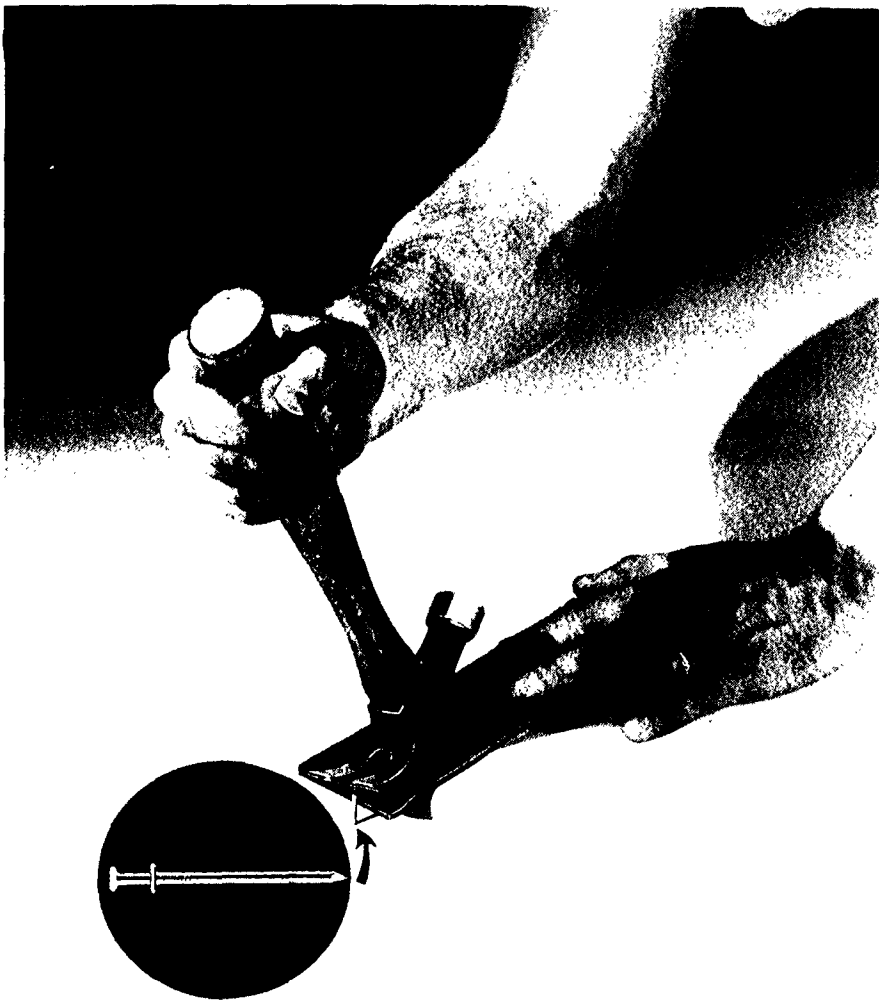
Fig. 48 Double-headed temporary nails are easily removed. A metal plate is used to protect the wallboard surface.
