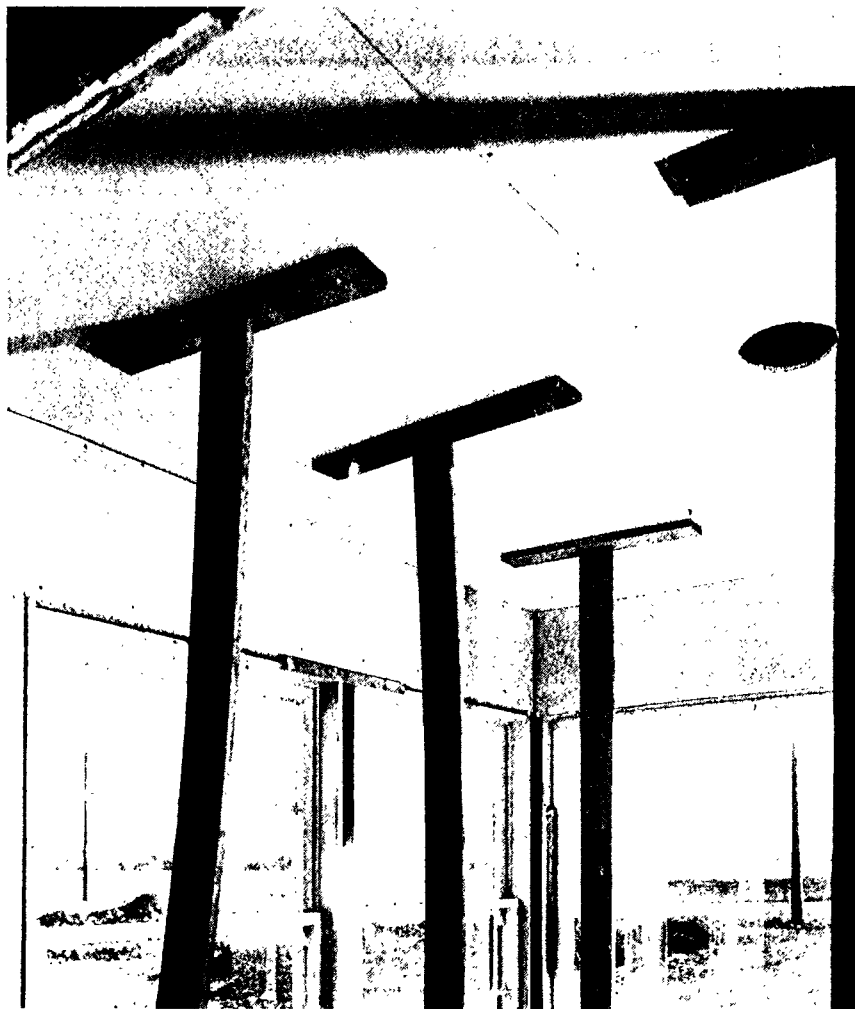
Fig. 39 Temporary bracing holds gypsumboard against supporting framing until adhesive bond develops.
