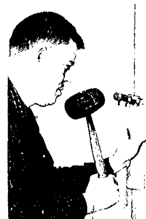
Fig. 61 Various tools are used to crimp cornerbead at the outside corner of gypsumboard facings on a column.
