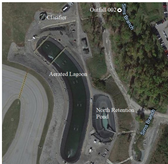
Figure 2. Overhead view of the Aeration Lagoon area.
