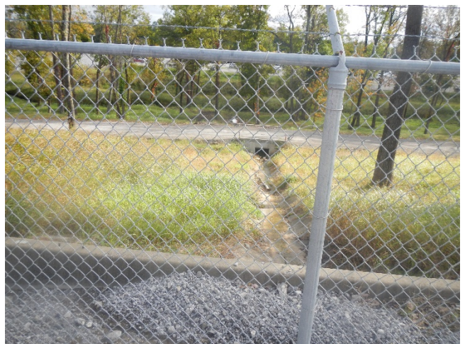
Photo 6. Open channel ditch to Outfall 002.
