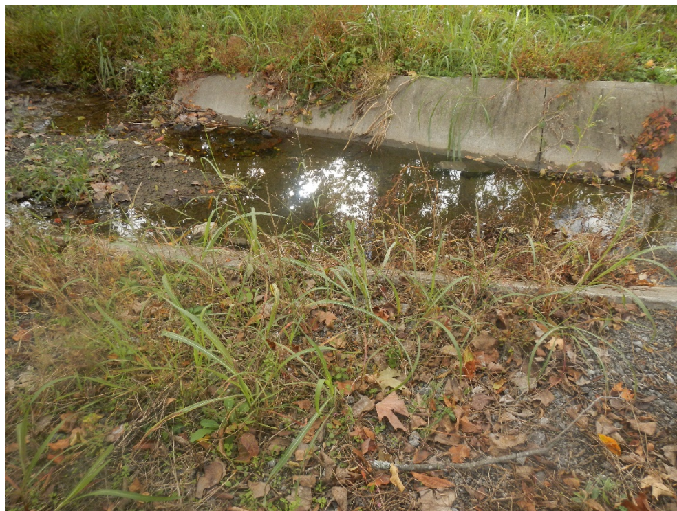
Photo 8. The end of the open channel ditch and sampling location for Outfall 002.
