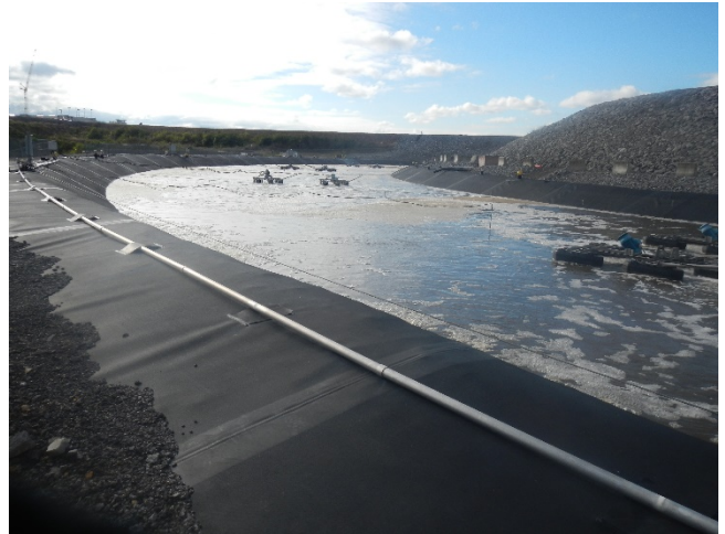
Photo 2. Aerated Lagoon, south section.
