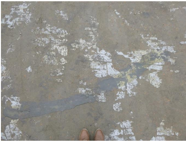
Photograph 13: Permitted Area 1 secondary containment.
