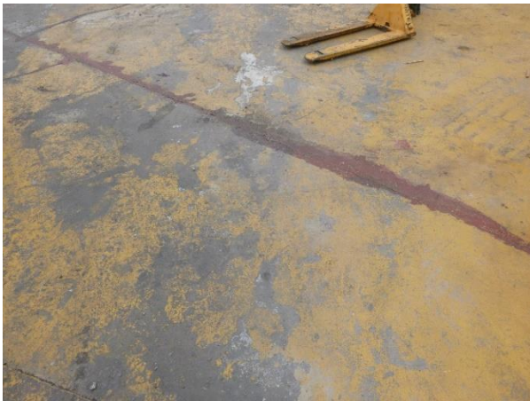
Photograph 14: Permitted Area 1 secondary containment.
