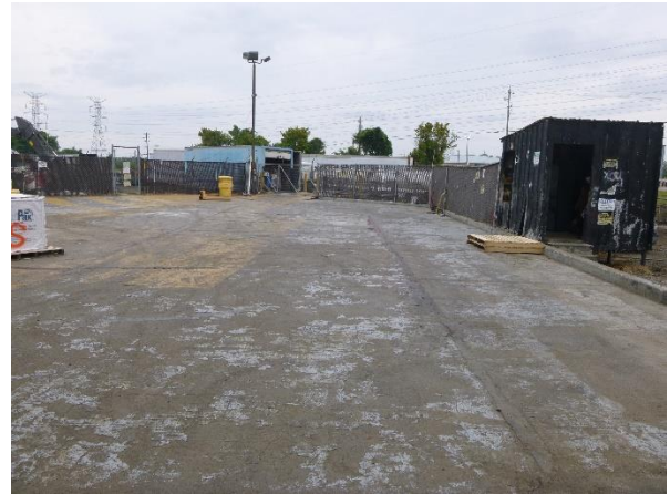
Photograph 10: Permitted area 1 - looking across Area 2, 3 and at 4 under the Shed.
