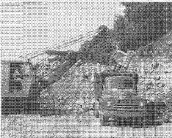
Revetment job nearing completion. All told, almost 250,000 tons of rock was put in place.
