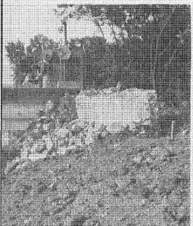
Bulldozer pushes stone in place to protect toe of the revetment.
