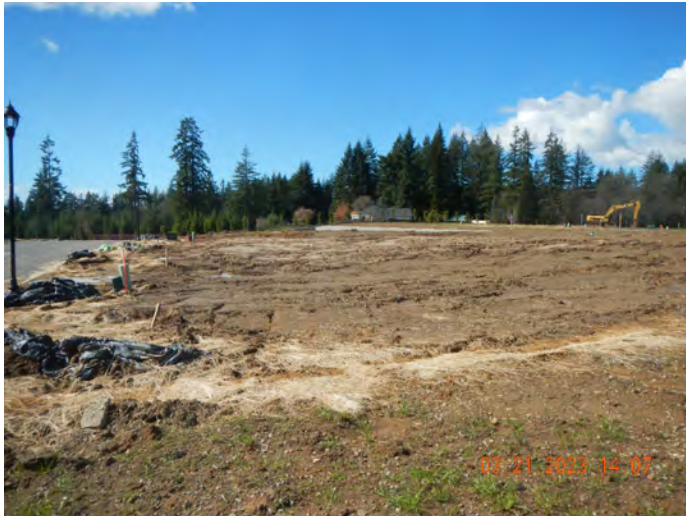
Photo #:11 (DSCN3190) Description: Facing west, photo of unstabilized areas within Phase 2. According to Mr. Hamilton, the stockpile was removed within the area the week prior.
