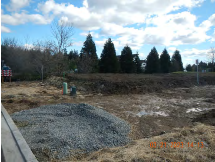
Photo #:13 (DSCN3192) Description: Facing east, photo of disturbed areas within the northeast corner of Phase 2.
