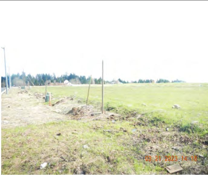
Photo #:15 (DSCN3194) Description: Facing east, photo of the north end of Phase 2. Photo taken from the northwest corner.
