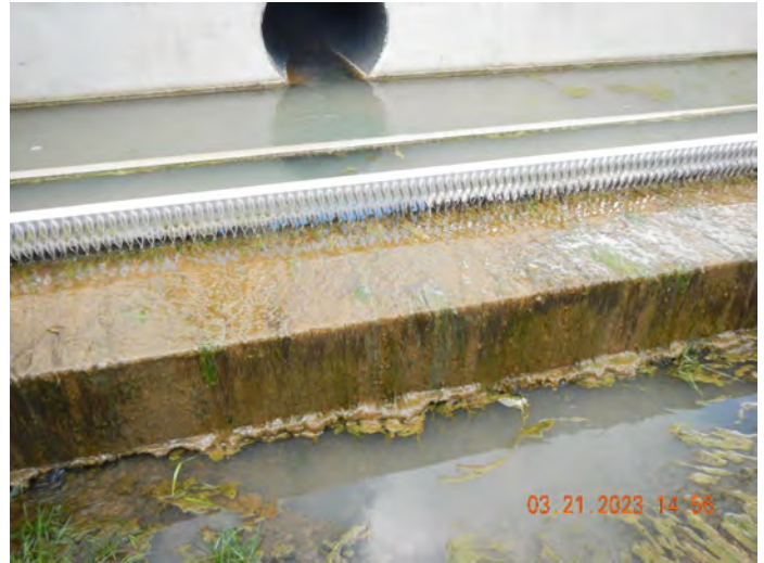
Photo #:20 (DSCN3199) Description: Facing north, photo of the constructed outfall from the stormwater pond to a tributary of Jenny Creek.
