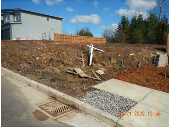
Photo #:09 (DSCN3188) Description: Facing northeast, photo of unstabilized lot (lot #52).
