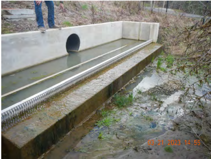
Photo #:19 (DSCN3198) Description: Facing northeast, photo of the constructed outfall from the stormwater pond to a tributary of Jenny Creek.
