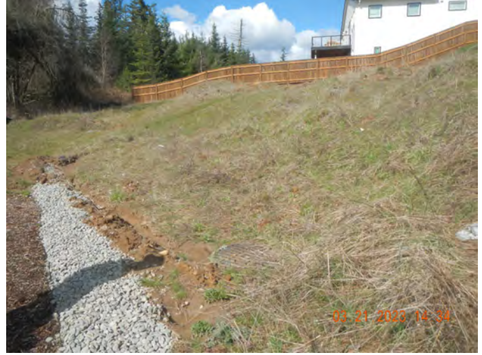
Photo #:18 (DSCN3197) Description: Facing west, photo of channeled drainage entering a constructed trench drain along the southwest perimeter of Phase 1.
