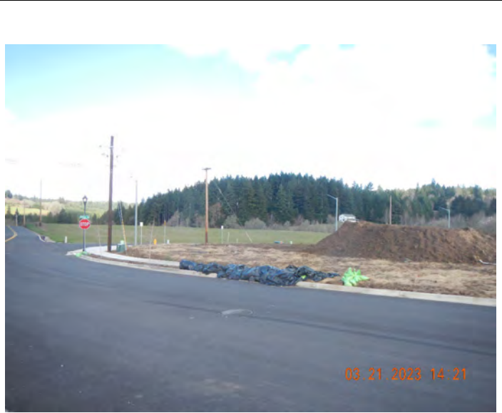
Photo #:14 (DSCN3193) Description: Facing south, photo of the northwest corner of Phase 2. Silt fencing was observed to be not extended to the corner.
