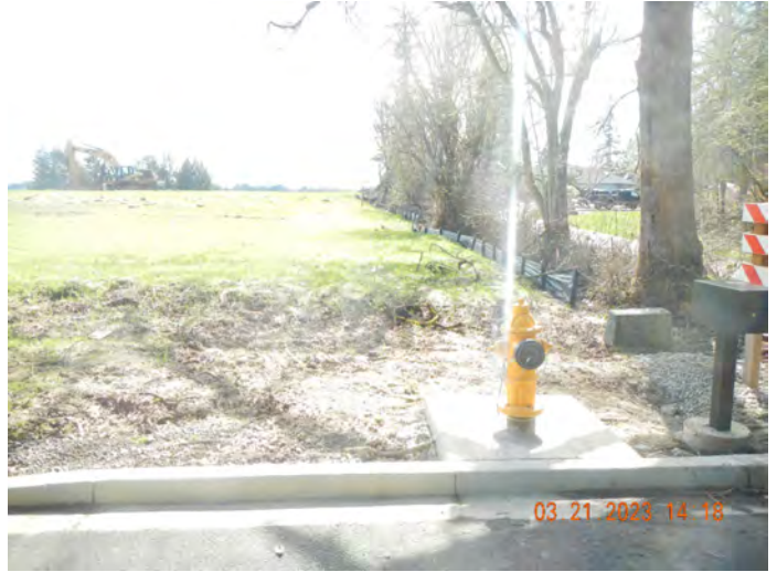
Photo #:14 (DSCN3193) Description: Facing south, photo of the northwest corner of Phase 2. Silt fencing was observed to be not extended to the corner.
