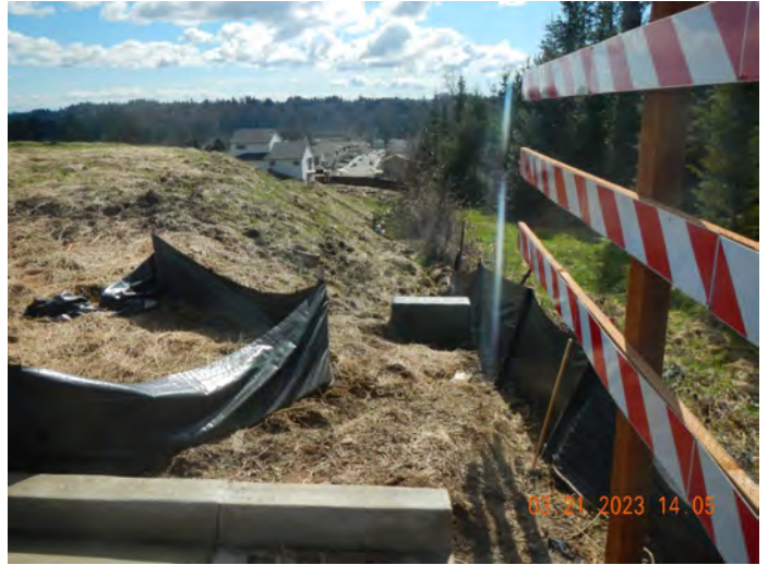
Photo #:10 (DSCN3189) Description: Facing south, photo of western perimeter within Phase 1.
