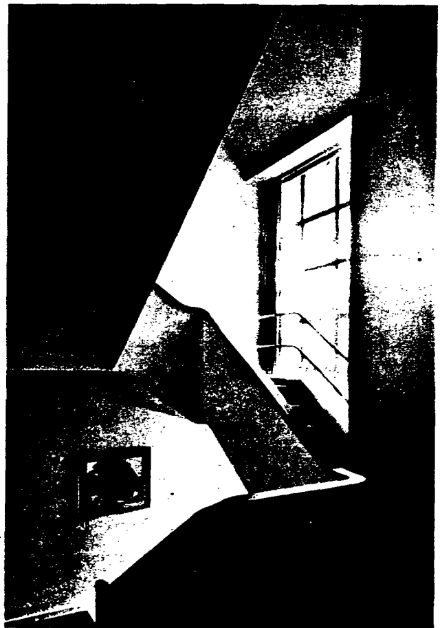
This staircase depends upon sheer form of structure for its beauty, and Red Top plaster over USC diamond mesh metal lath make this conception of beauty a possibility. Lights and shadows from the big window provide all the ornamentation.
