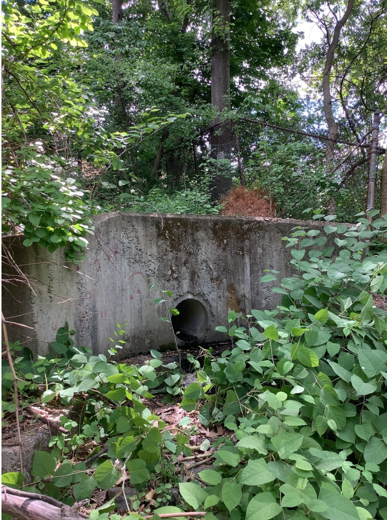
French (photo taken 5/24 at 12:05 PM): Outfall located at the eastern corner of the parking lot behind the church on All Saints Lane. Flow was a trickle into the Spickett River. No sample was collected at this location.
