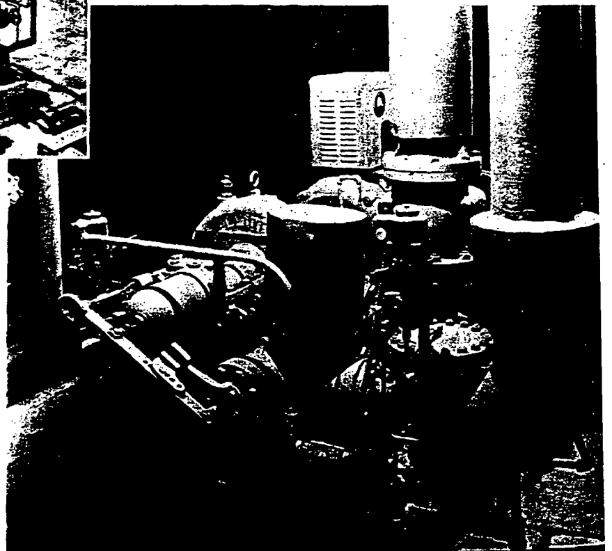
Mounted on the generator is the built-in control. In the housing is the voltage regulator and control panel.
