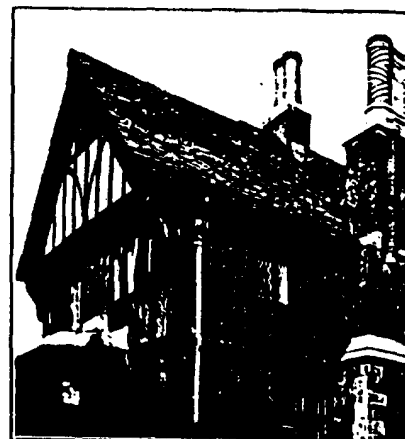
A half dozen uses for lead on this house—gutters, leader-heads, downspouts, flashing, bay window roof, sun-dial, and leaded windows.
