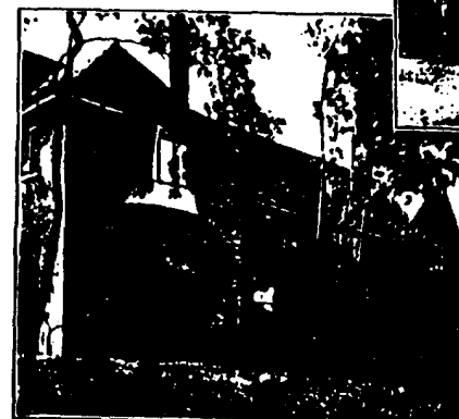
A lead-roofed bay window and leaded windows blend pleasingly with the architecture of this modest home.
