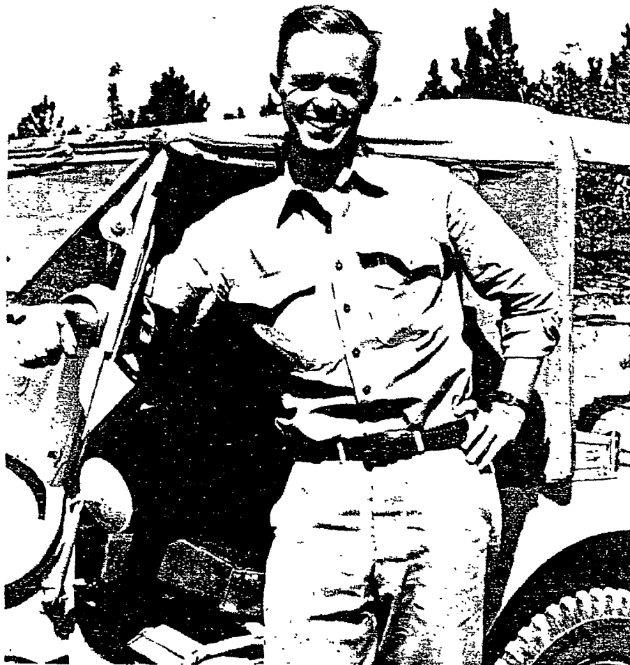
Steve Bechtel, Jr., pipe liner.
