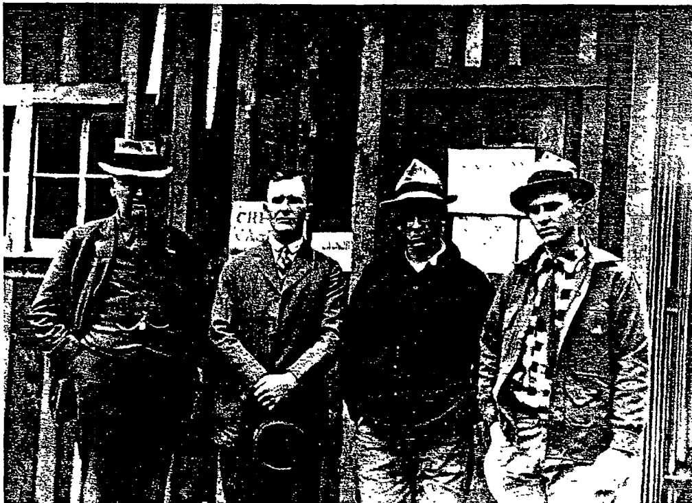
Railroad builders—Dad and the boys during construction of the Natron Cut-Off.
