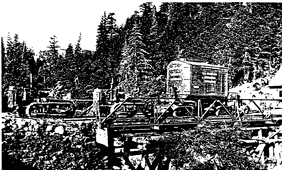
Shoring-up a bridge to withstand heavy loads. As equipment grew larger, the problems of transporting it multiplied.
