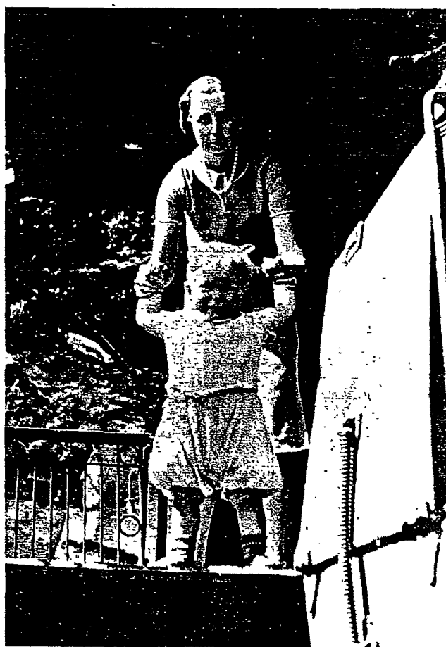
Mrs. W. E. Waste with Steve, Jr., third generation constructor, at Natron Cut-Off
