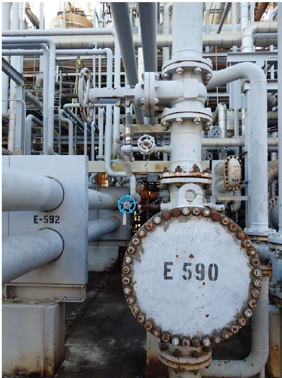
Photograph 12 - File: PB140012.JPG Overview of Exchanger E-590.
