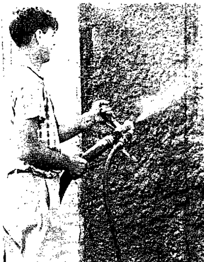
● NOZZLEMAN SCRATCHING metal lath with True Gun-All
