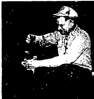
SAMPLES PAINT: Cheesecloth keeps impurities out of test. Mixing varies from 20 to 60 hrs. at 100 to 150 depending on formula.
