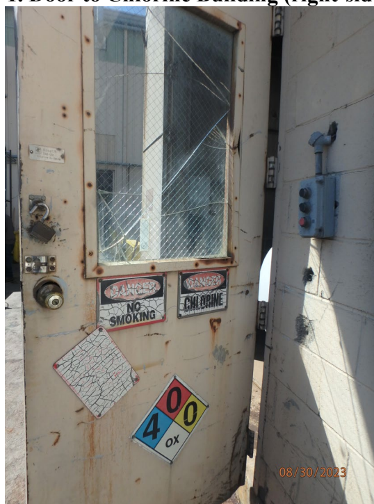
Photo 1. Door to Chlorine Building (right-side door)
