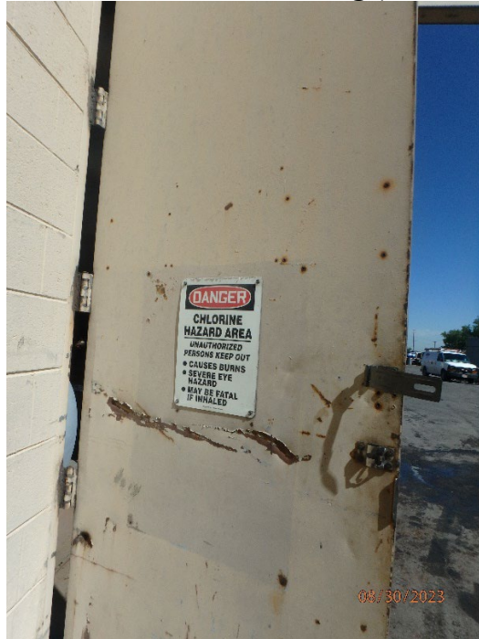
Photo 2. Door to Chlorine Building (Left side door)
