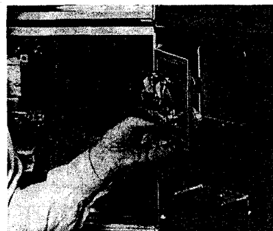
Unit Withdrawal Facilitated by Removable Operators Panel—No Push Button Wires to Be Disconnected.
