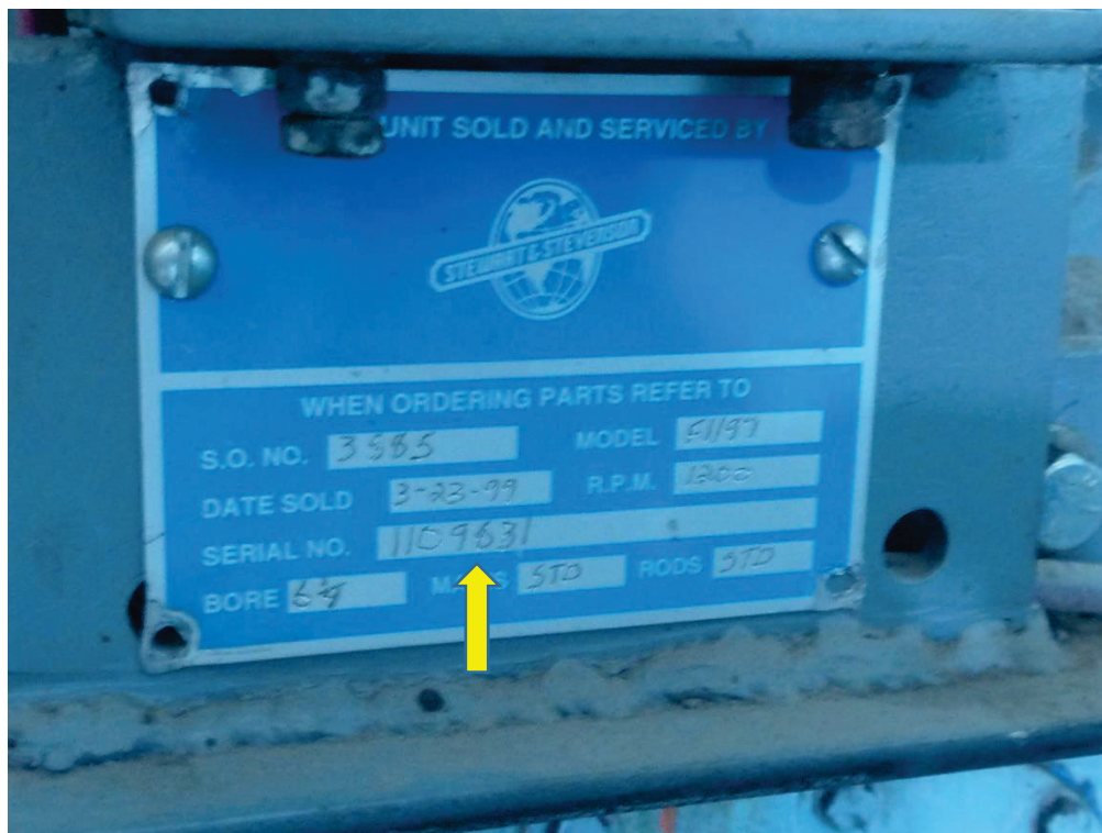
Faceplate of Waukesha F1197G, 100 kW Generator Set with Serial Number: 1109831 (emphasis added)
