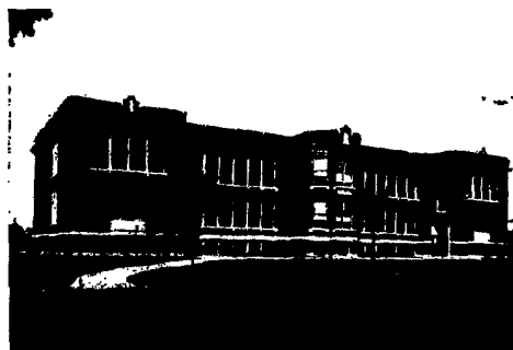
Jackson School Building, Cedar Rapids, Iowa. S-W, ODP and Flat-tone were used for finishing materials
