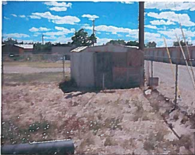
PRESSURE TANK BUILDING
