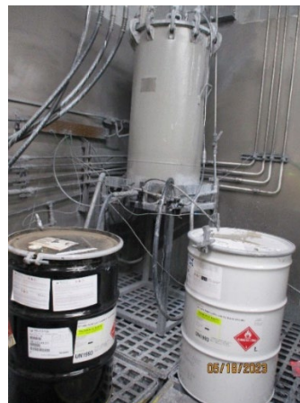
Photo 14: Two (2) 55-gallon drums of paint line flushing (from two different paint lines), properly closed, labeled “Hazardous Waste”, and marked with an indication of hazard.
