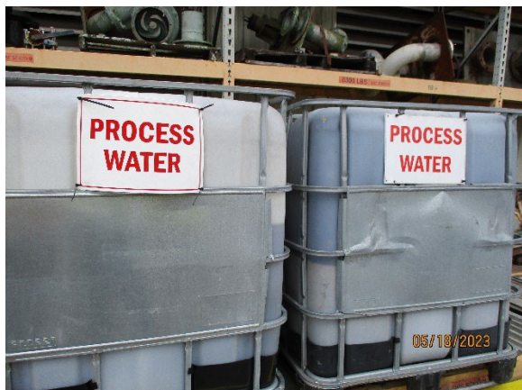
Photo 25: Used Oil Storage Area 2 for oily water. Inspectors recommended re-labeling the containers to “Oily Water” instead of process water.
