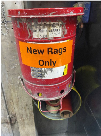
Photo 29: New label for red container in Paint Room (in between paint booths) for new rags only.
