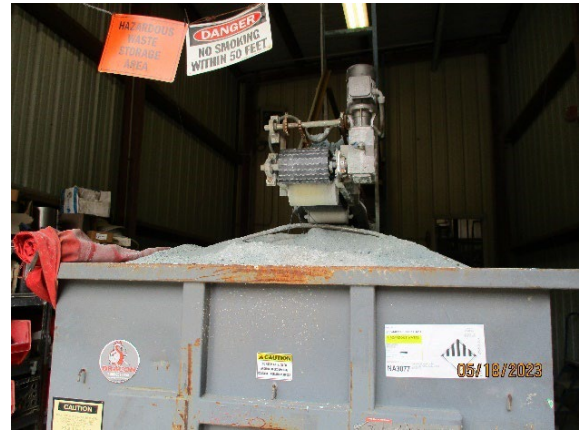
Photo 20: Filter cake being added to hazardous waste roll off container in WWTP.
