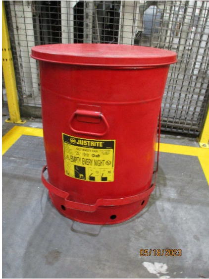
Photo 5: 5-gallon red container labeled “Oily Waste Can”.
