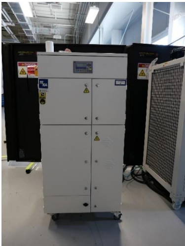
Photograph #7 – Lab 2651 SAA containers.
