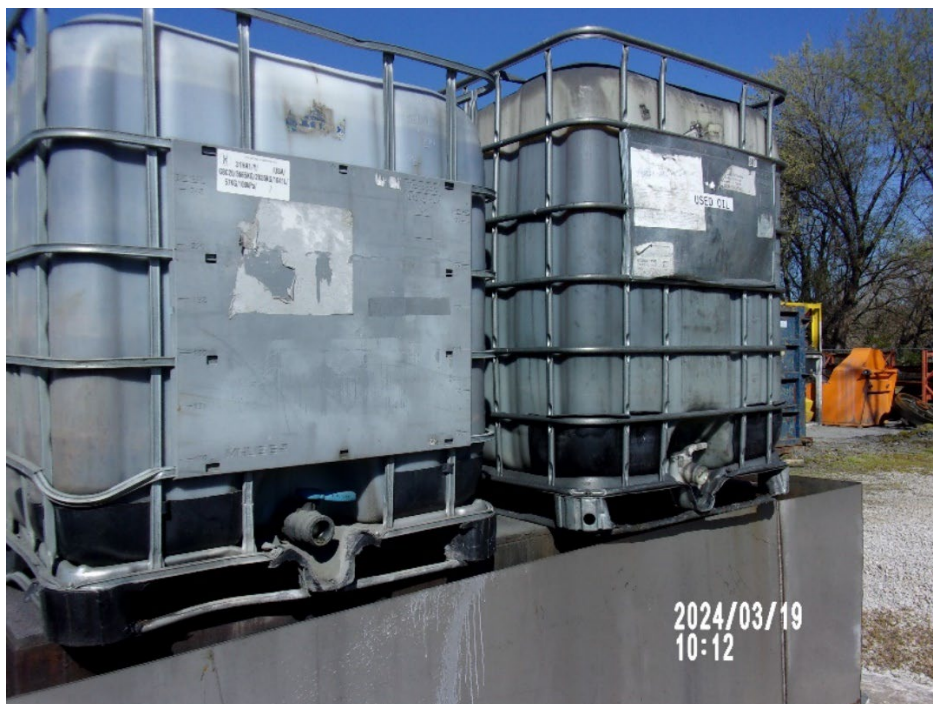
Photograph 7: Picture of Used Oil Containers Above Secondary Containment. One container Is Missing the “Used Oil” Label.
