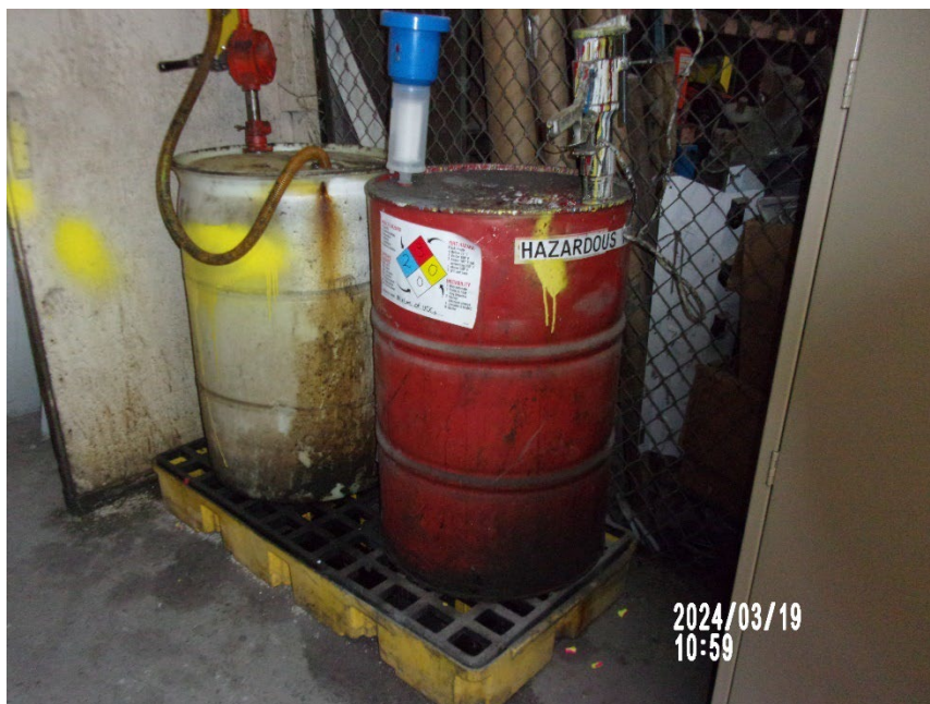
Photograph 10: Hazardous Waste Satellite Accumulation Container. Container is Labeled as Hazardous Waste and has a Hazard Marking.
