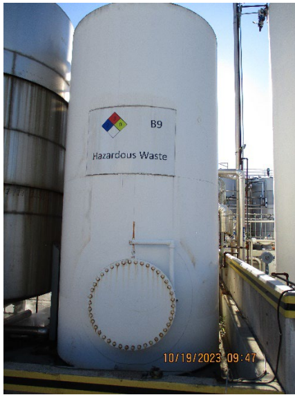
Photo 5: Hazardous waste Tank B-9.
