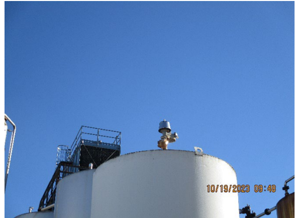
Photo 6: Top of Tank B-9.
