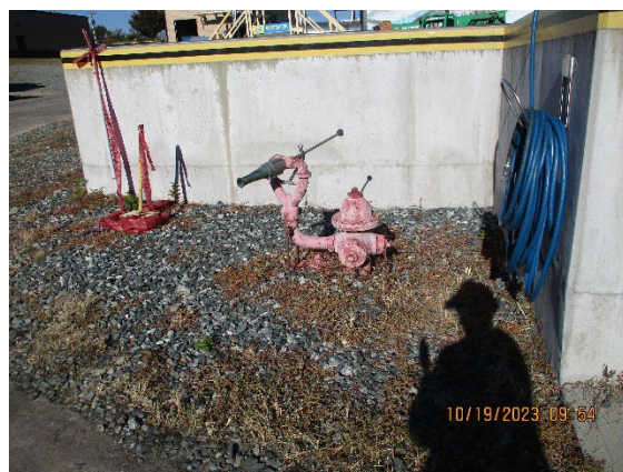
Photo 4: Fire hydrant next to B-Tank Farm.
