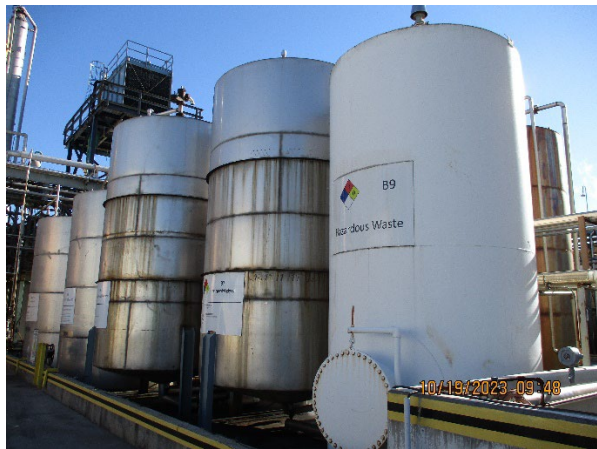
Photo 7: Hazardous waste Tank B-9.
