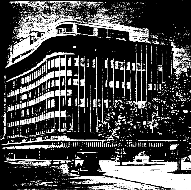
Store of Peter Jones, Ltd., London, on which lead flower boxes at the second and sixth floors are unusual and attractive architectural features.
